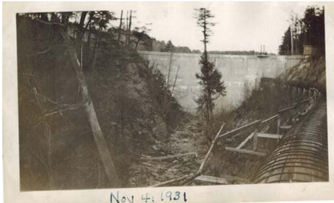
The old penstock at the dam, courtesy of the Marlborough Historical Society
