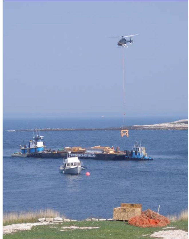
The helicopter used to transport the timber.
