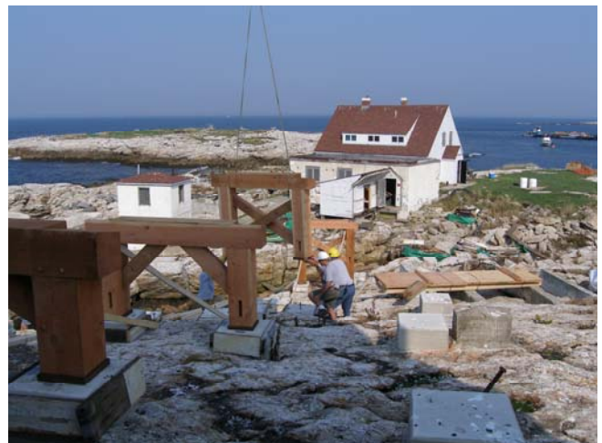
Setting the timber trestles.
