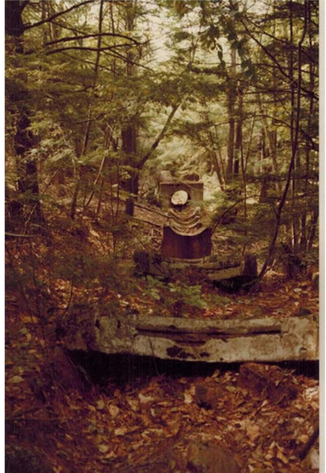
The concrete penstock cradles, Ed Goodrich
