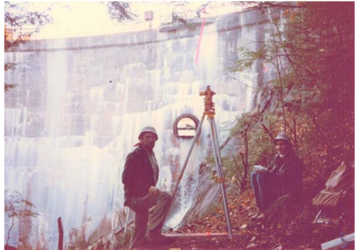
Ed & Gilda surveying the penstock in the gorge, Ed Goodrich
